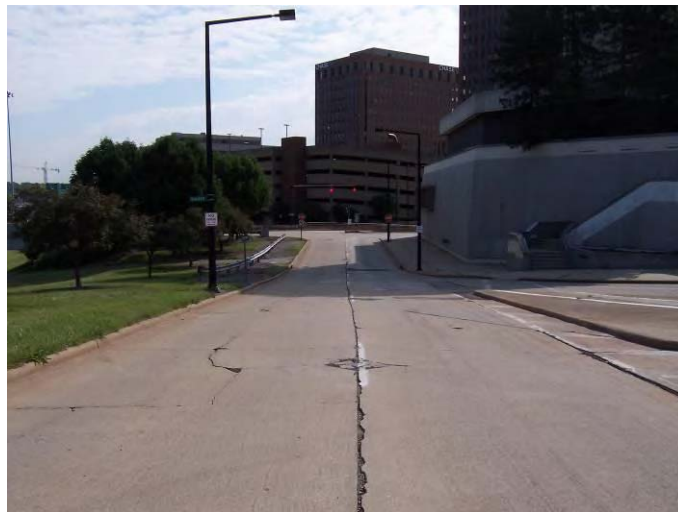
Photo 1. Looking north along Dart Avenue toward Mill Street intersection.
